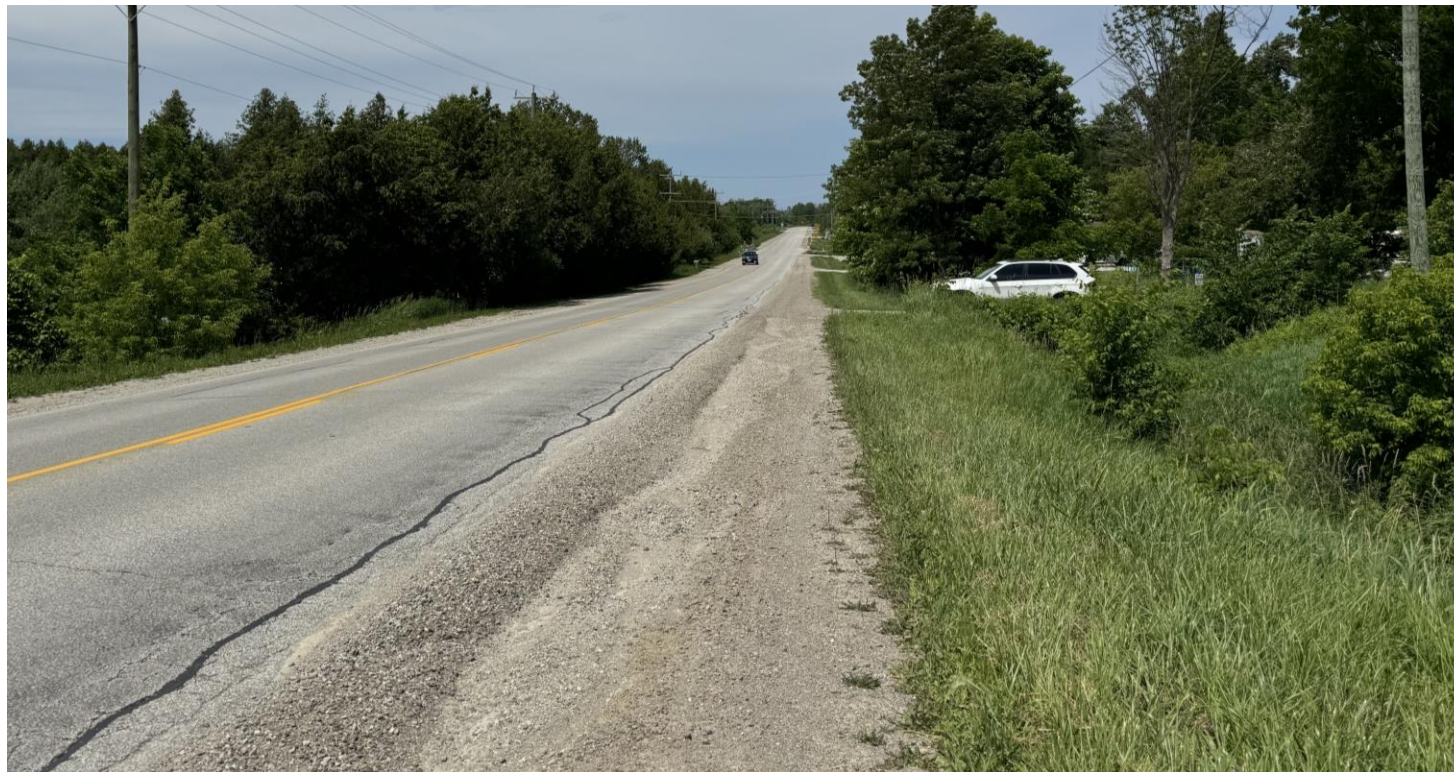
Looking north along Grey Road 2 from site access
