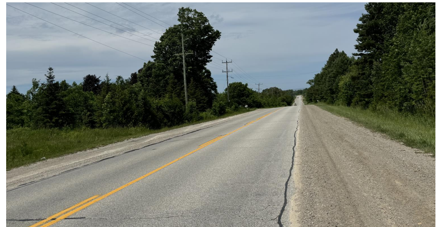
Looking north along Grey Road 2 towards site access
