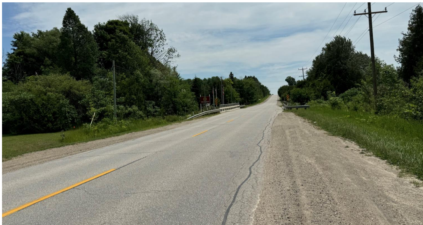
Looking south along Grey Road 2 towards site access
