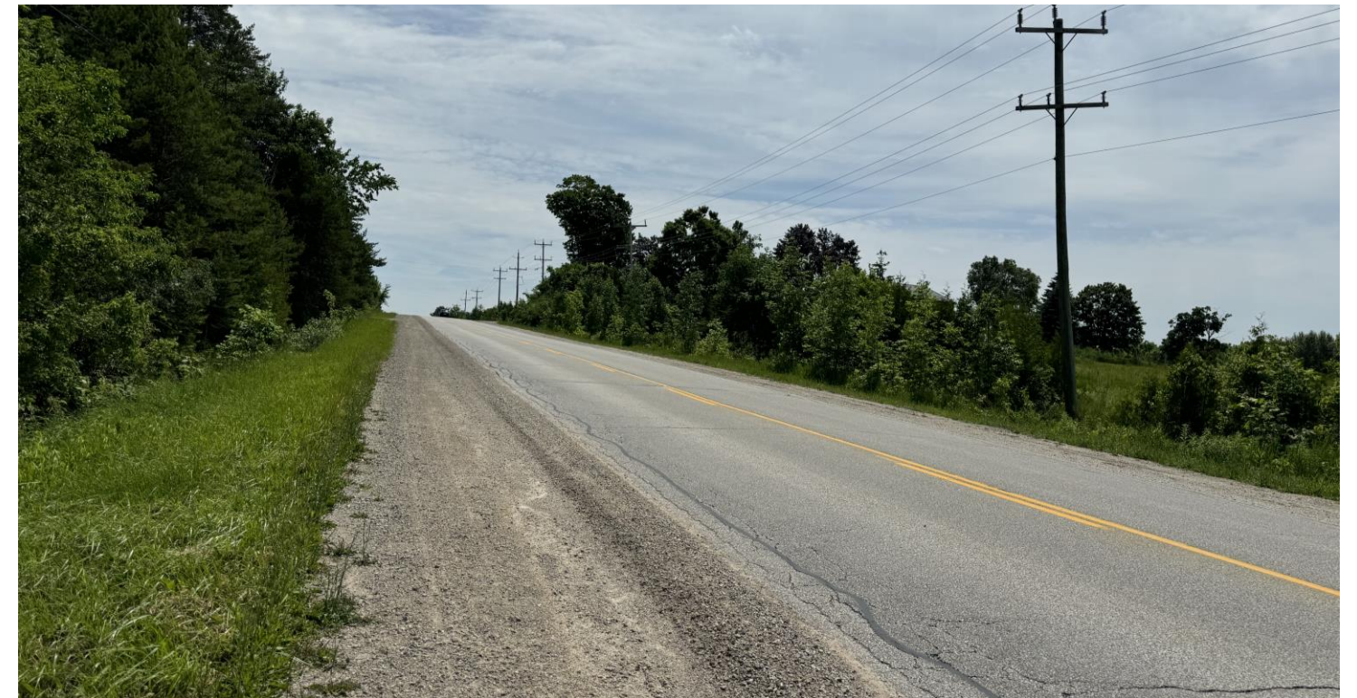
Looking south along Grey Road 2 from site access
