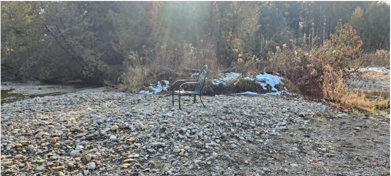
Photo P4: Slope and creek conditions in area of Sections X3-X3 to X4-X4 (looking south)
