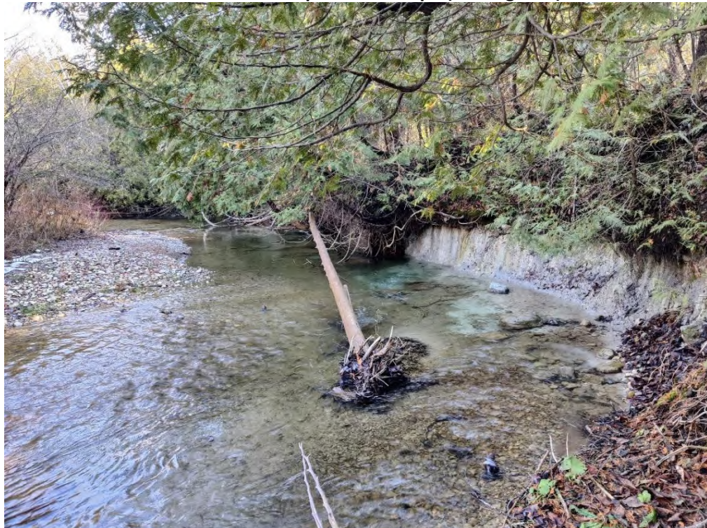
Photo P10: Creek and slope conditions in east part of site near Section X13-X13, with Erosions at lower portion of slope (looking east)
