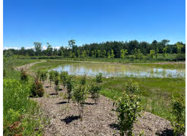
Figure 18. Stormwater Management Facility Planting.
