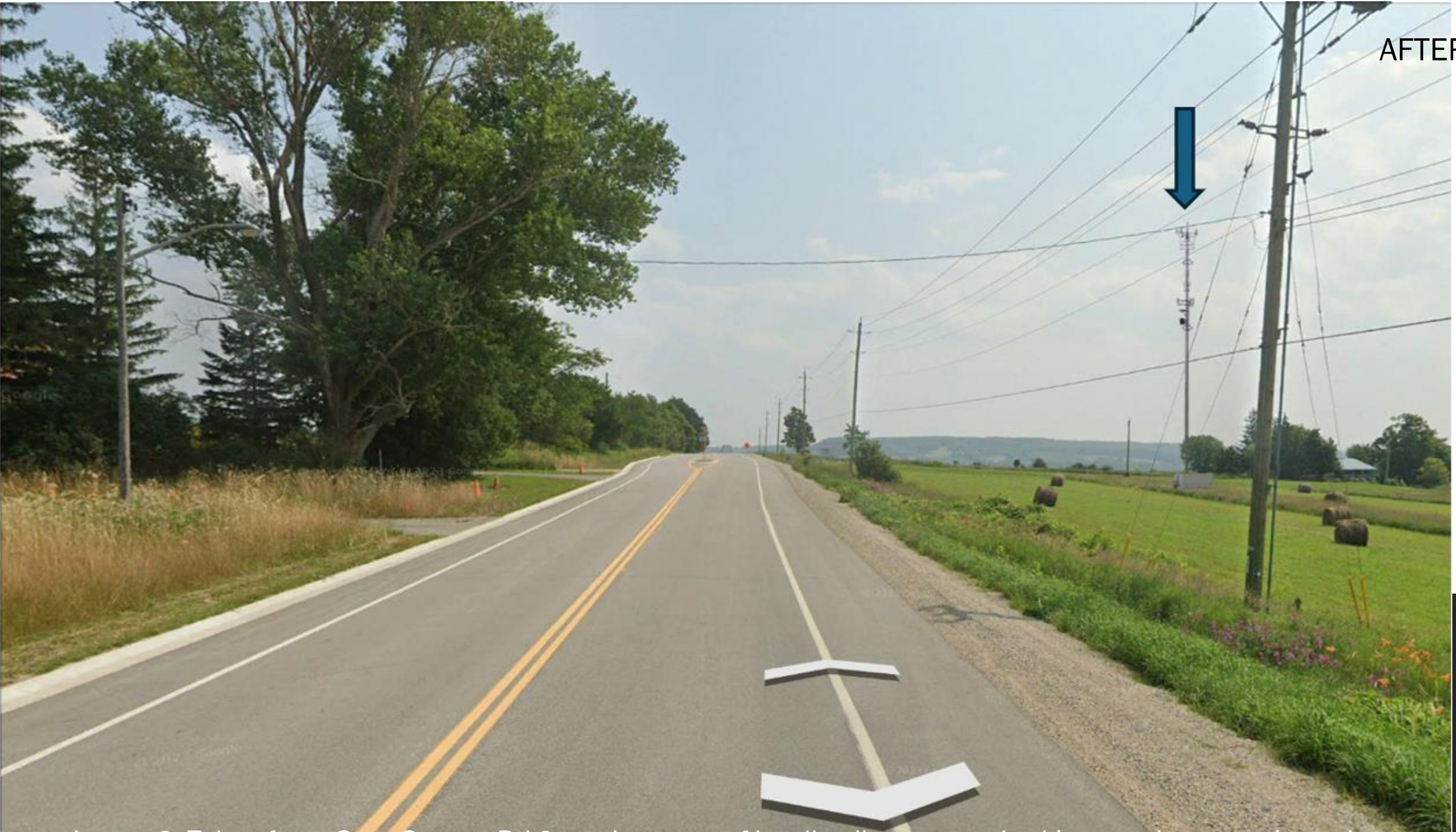
Image 2: Taken from Grey County Rd 2 north corner of landlord's property looking south, approximately 350m from proposed site, showing potential equipment from multiple carriers
