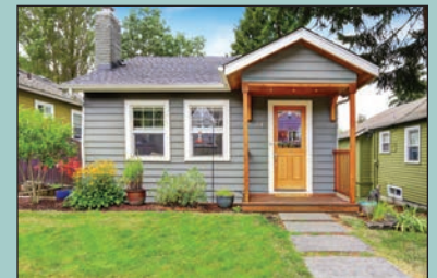
Figure 2: A site-built tiny home
