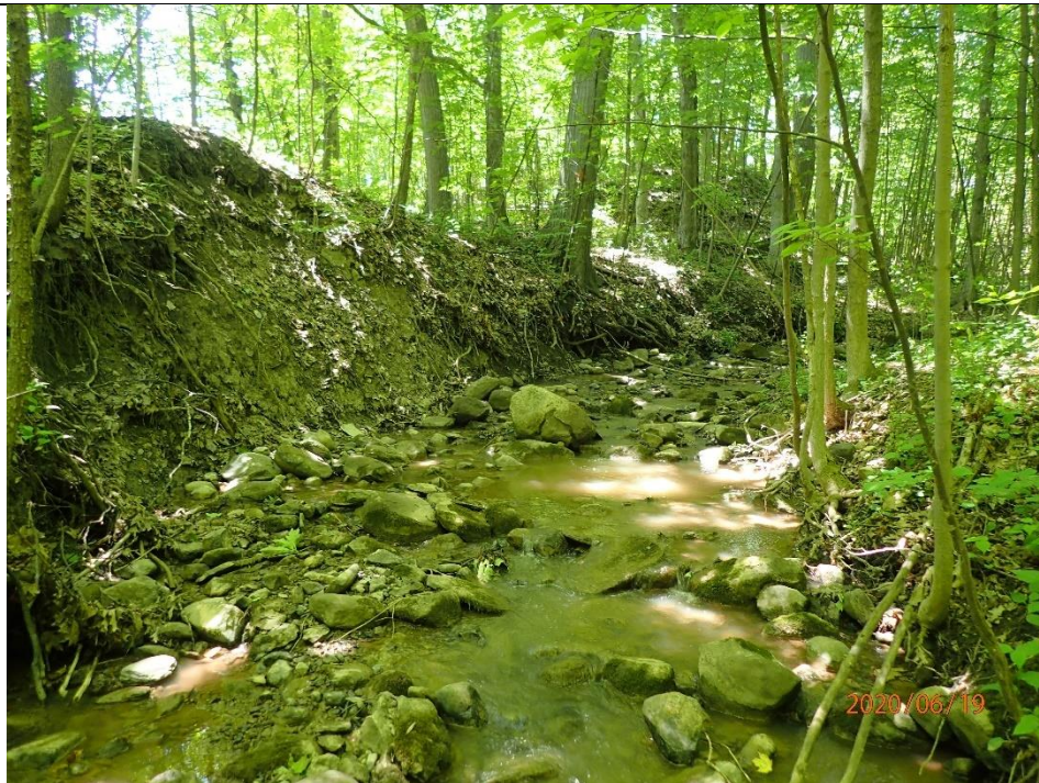
Bank failure was present along outside meander bends. Undercuts up to 0.9 m were observed and exacerbated by leaning tree root systems.
