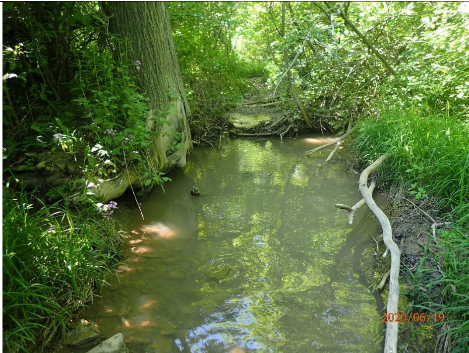
Bank erosion was present through 30 to 60% of the reach and was observed through scouring of the channel banks. Basal scour was observed along more than 50% of total length.
