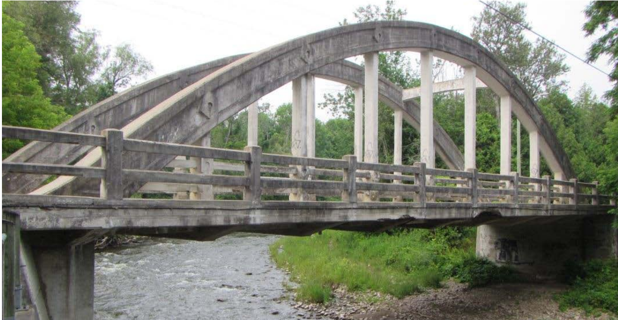
Photo #1: Black Bridge Structure
