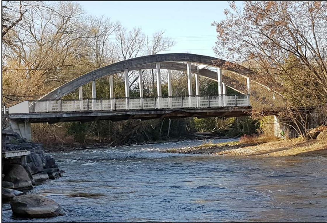
Photo #2: Black Bridge with vertical metal sections
